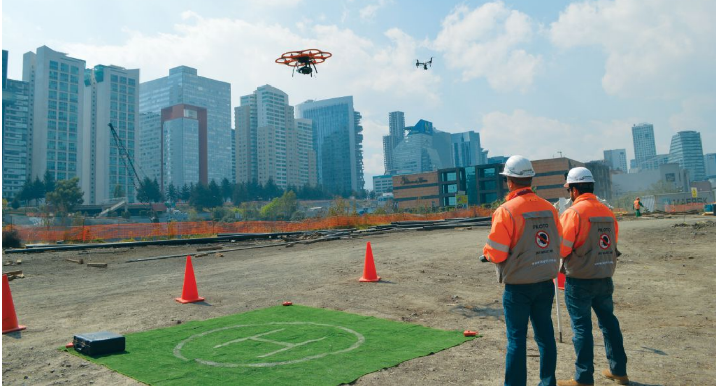
Drones were used from the beginning of the project with various payloads, including a DSLR camera.
