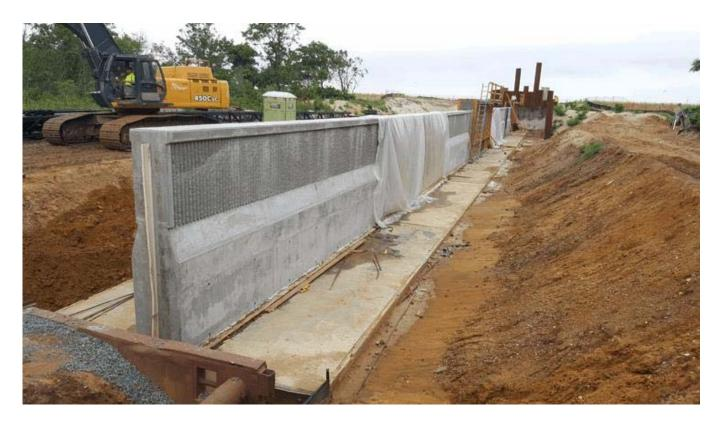
A concrete floodwall is being constructed to help reduce flooding. (Credit: JoAnne Castagna, Public Affairs)
