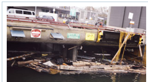
Hurricane Sandy flooded the Battery Park Underpass, which keeps traffic flowing independently of the labyrinthine streets that make up the southern tip of
