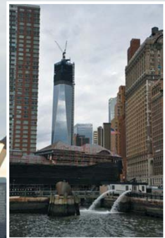
Some of an approximate total of 57 million gallons of water is pumped out of the Battery Park Underpass just days after Sandy hit as part of the U.S. Army Corps of Engineers’ unwatering mission. (Photo by Chris Gardner, New York District public affairs)
