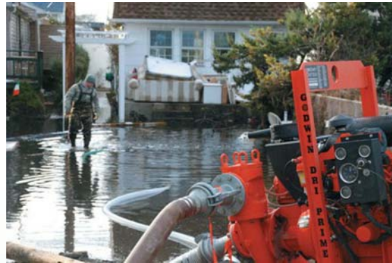
Members, supporting the Army Corps FEMA mission to allow access to flooded homes in Breezy Point, N.Y., pumped an average of 750,000 to 1 million gallons of water a day in the week following Hurricane Sandy. (Photo by Mary Markos, St. Louis District, public affairs)
