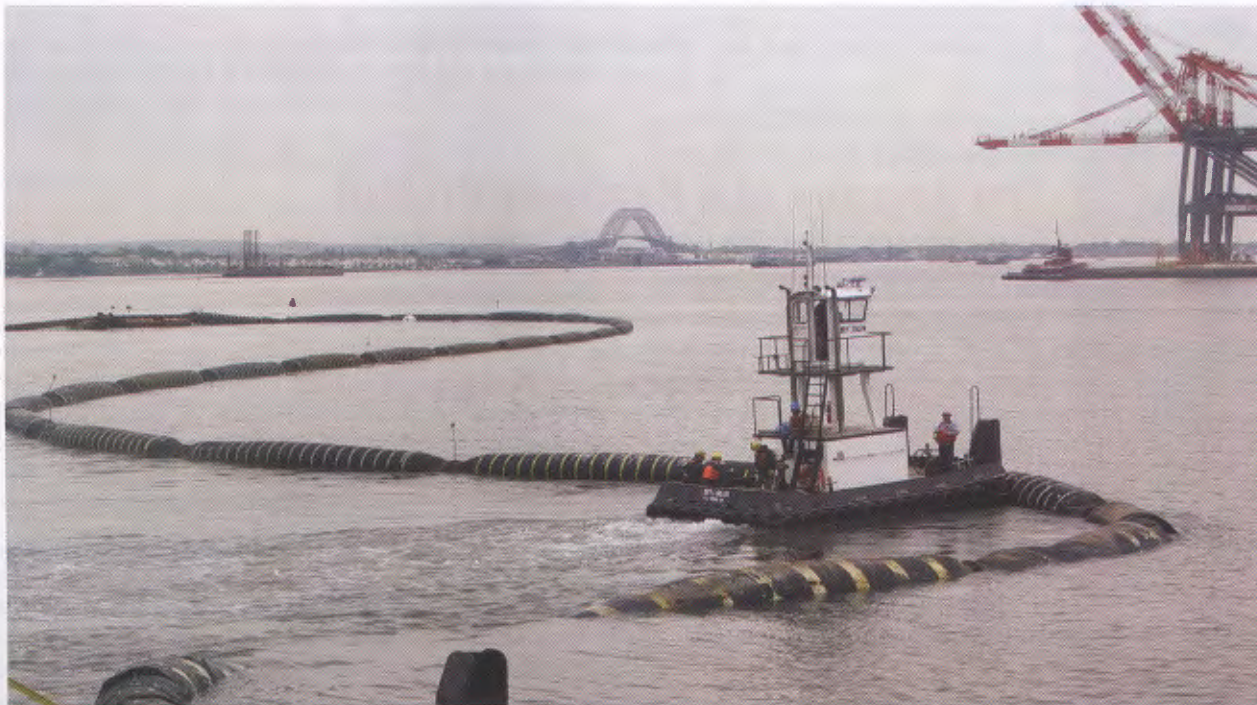
Dredged sand was used to cap the Newark Bay CDF. A floating pipeline connected the dredge to the pump barge at the CDF site. Photo: Linda Guenther, U.S. Army Corps of Engineers
