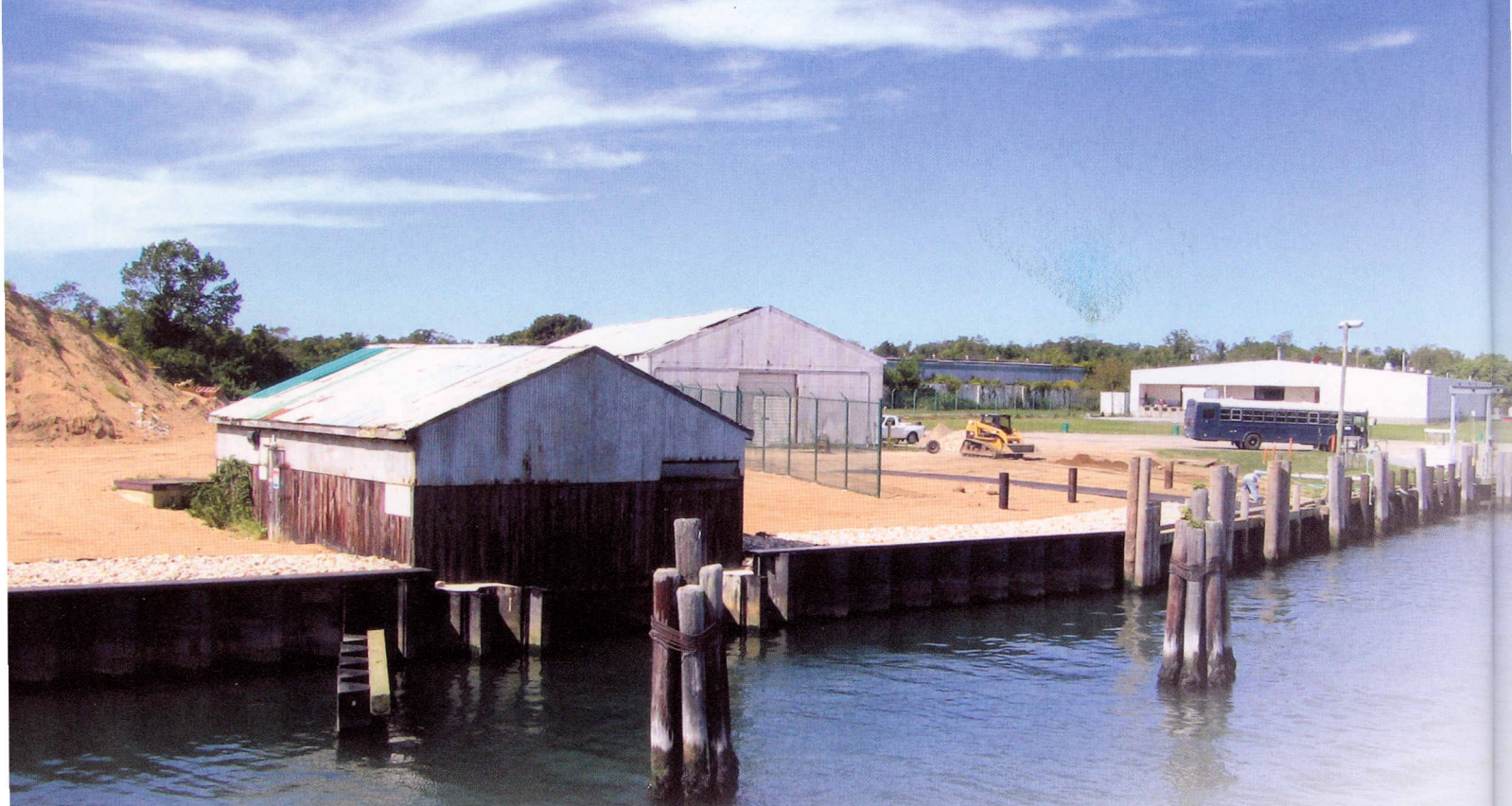
Restored bulkhead on Plum Island
