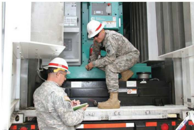
In Rockaway, Queens, NY, Staff Sgt. Henry Howell and Sgt. Nathaniel Boecker of Headquarters and Headquarters Company, 249th Eng. Battalion (Prime Power), inspect generators at the Ocean Bay Public Housing complex. The 249th has installed 22 generators powering 24 family building structures in the Rockaways.
